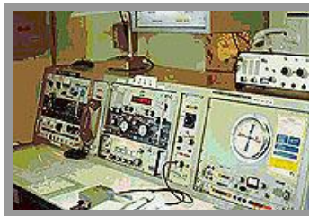
Figure 4: Typical merchant ship radio room - mid 1980's 4
