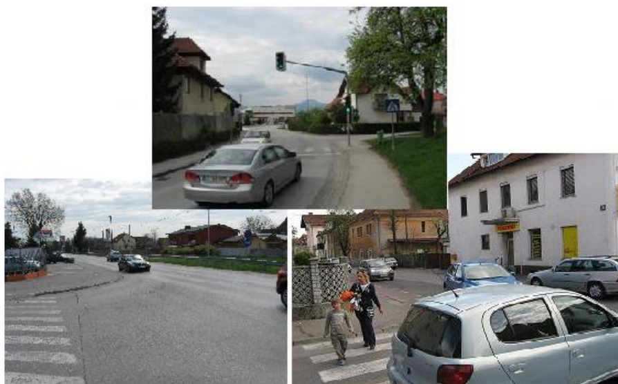
Figure 6: Accident spots: inadequate visibility angle, connection to main road in curve (combine with high speed in main road)
