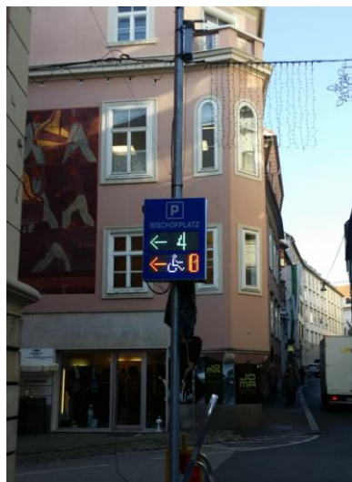
Figure 6: Electronic street PGI panel and communication interface on a public lighting pole [6]
