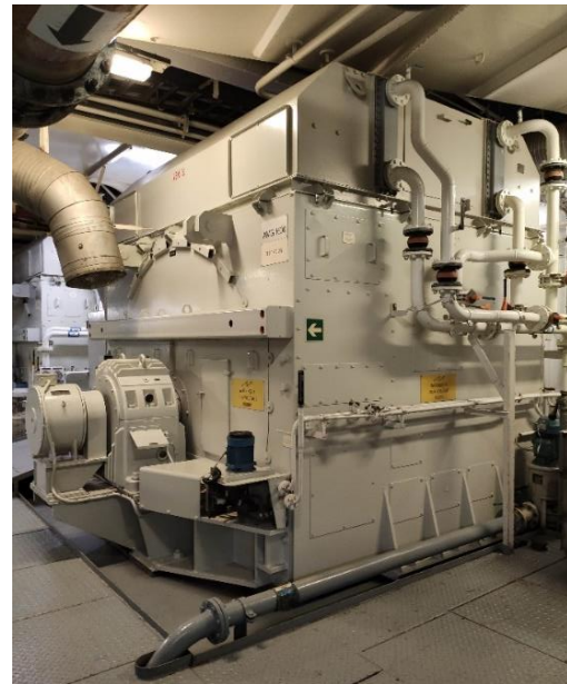
Figure 1: Synchronous generator
